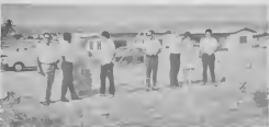
Board members and members of Aruba Amateur Radio Club (l to r in left picture) J. H. Hassell, M. Angela, J. Geerlings, H. Schenkel, C. C. Liefers, Mrs. Liefers and J. Noguera inspect progress of construction on their new clubhouse near Casa Cuna on May 4. Picture at right was taken a few weeks later.
